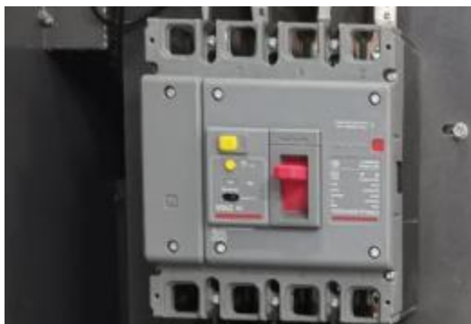
1. Bottom Circuit breaker "ON"
