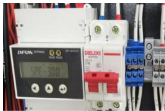
2. Intermediate air switch "ON"
