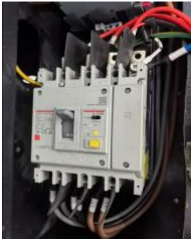
1. Bottom Circuit breaker "ON"
